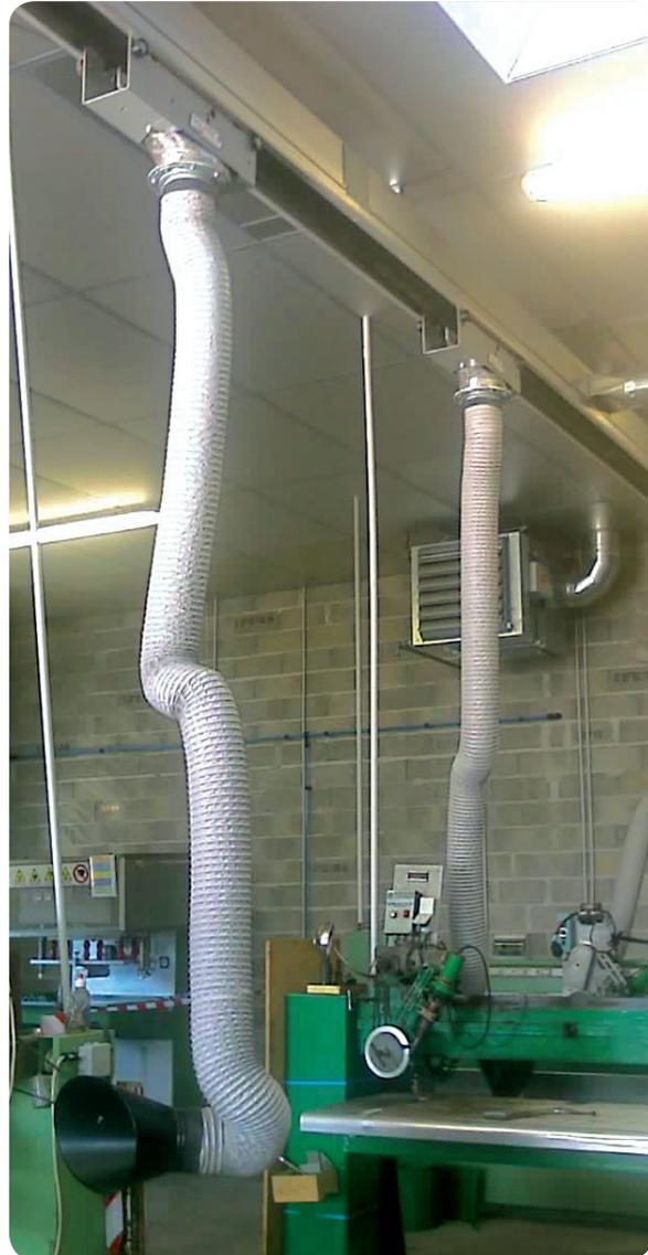
Aspiration sur machine outil/Aspiration on tool machine
