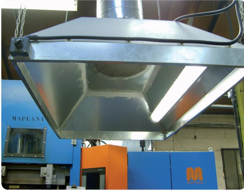
Hotte d'aspiration poste de moulage/Exhaust capture nozzle for moulding station
